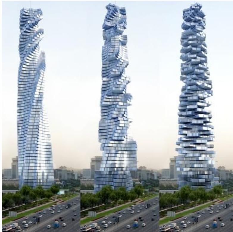
The rotation takes up to 3 hours (so you're not always spilling your coffee), and gets power from photovoltaic solar cells and 79 wind turbines, one located between each floor. The system is meant to create enough energy to power to the entire tower and still have juice to spare for some surrounding buildings. According to Fisher, two of these \$700 million futuristic scrapers are planned so far, one each in Dubai and Moscow. They will be built using a truly radical technique.
